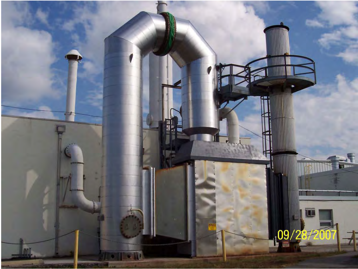
TFO before demolition.
