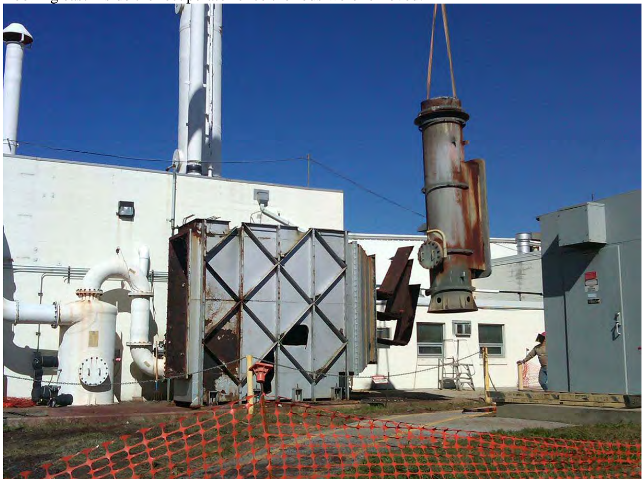
View of the east stack of the TFO (effluent side) being lifted off.
