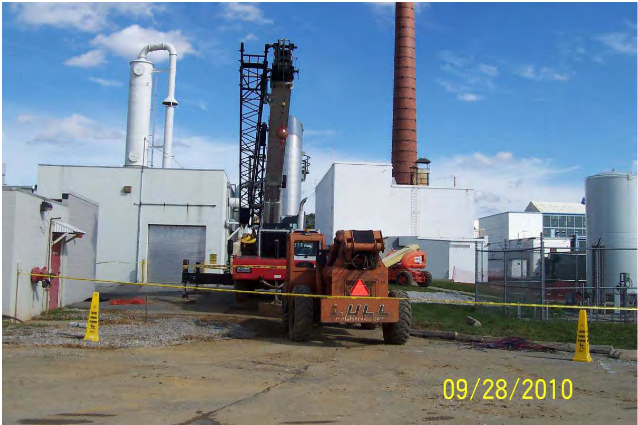
Crane used to lift stacks.
