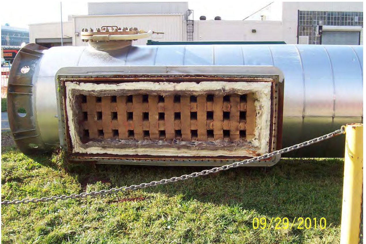
TFO western stack lying on the ground looking at the refractory bricks.
