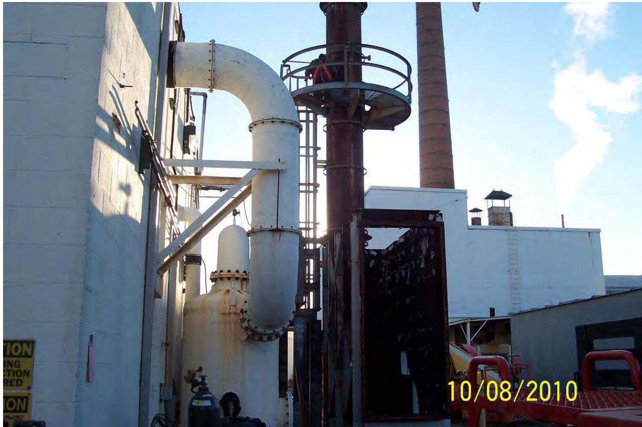
Looking east inside the recuperator once the rods were removed.
