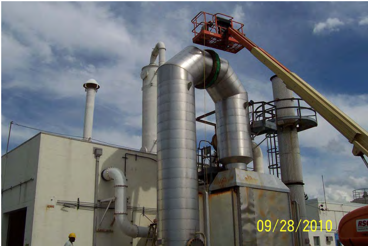
S&T removing the bolts in the flexible joint.
