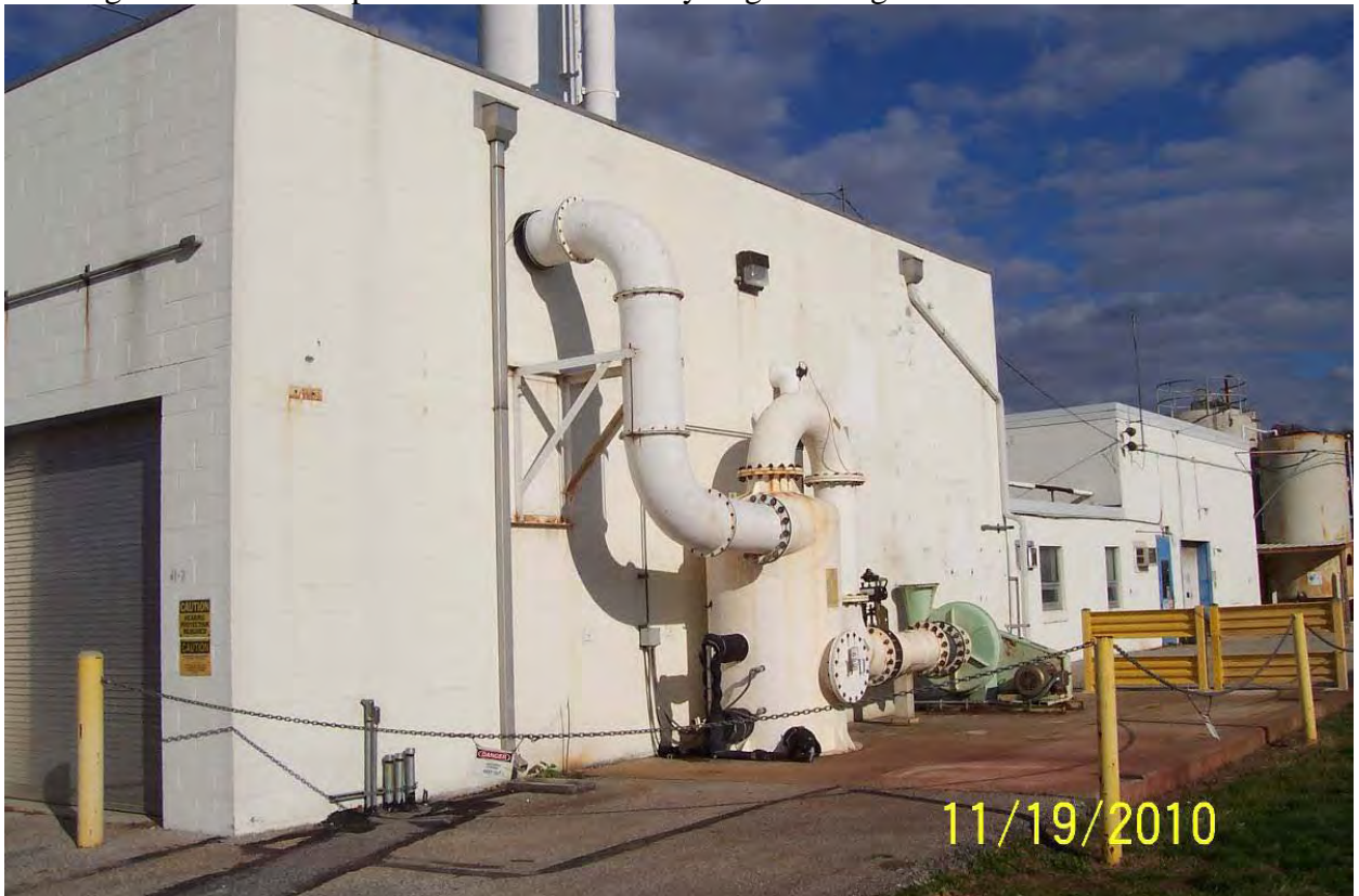
Looking northeast at the TFO pad after the TFO was removed.
